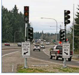
**Adaptive Signal Expansion**: (\$600k CMAQ) This project consists of improvements in the Salmon Creek and Hazel Dell areas as the next step in the operation and expansion of adaptive signals in Clark County.
