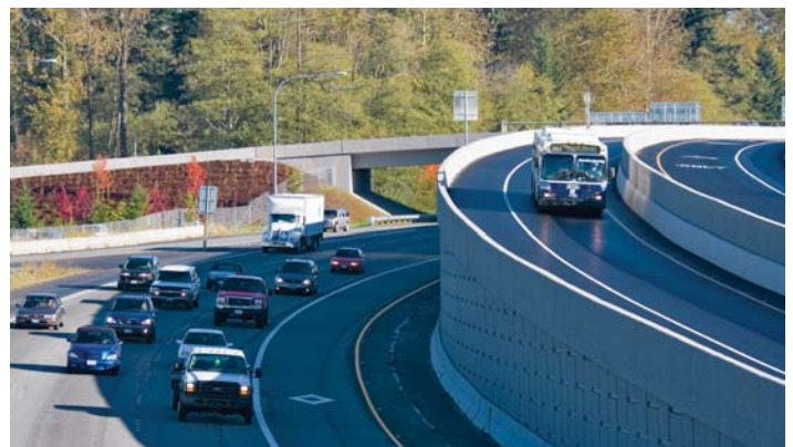
Exclusive Bus Ramp in Puget Sound
